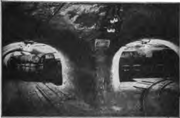
VIEW OF SUBWAY OF ILLINOIS TUNNEL CO.
